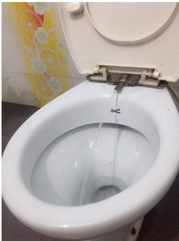
**Figure 1.** Water Emanating as a Single Stream form a Nozzle at the Back End of the Toilet Commode
